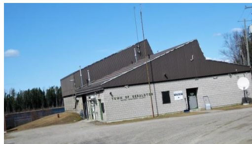
Water Treatment Plant - Geraldton
