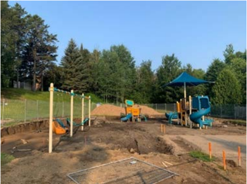
Wasco Park Playground, Thunder Bay (under construction)
